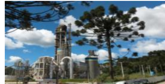
Continuous emissions monitoring
