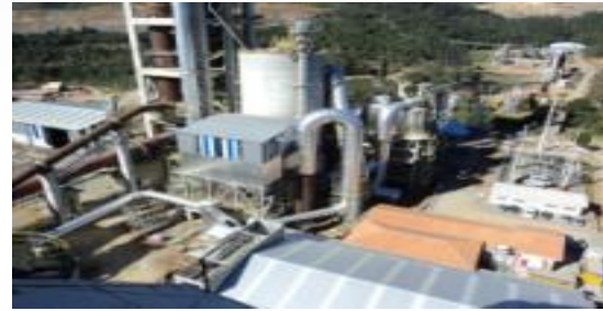
SNCR system for NOx abatement
