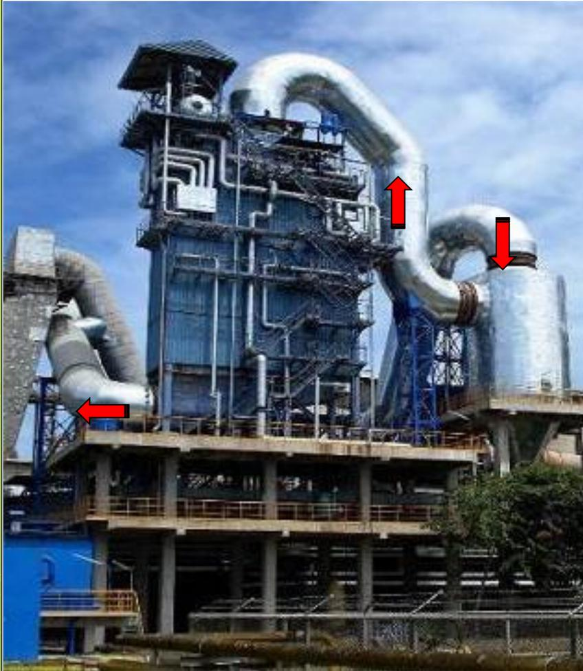
Separate Settling Chamber
