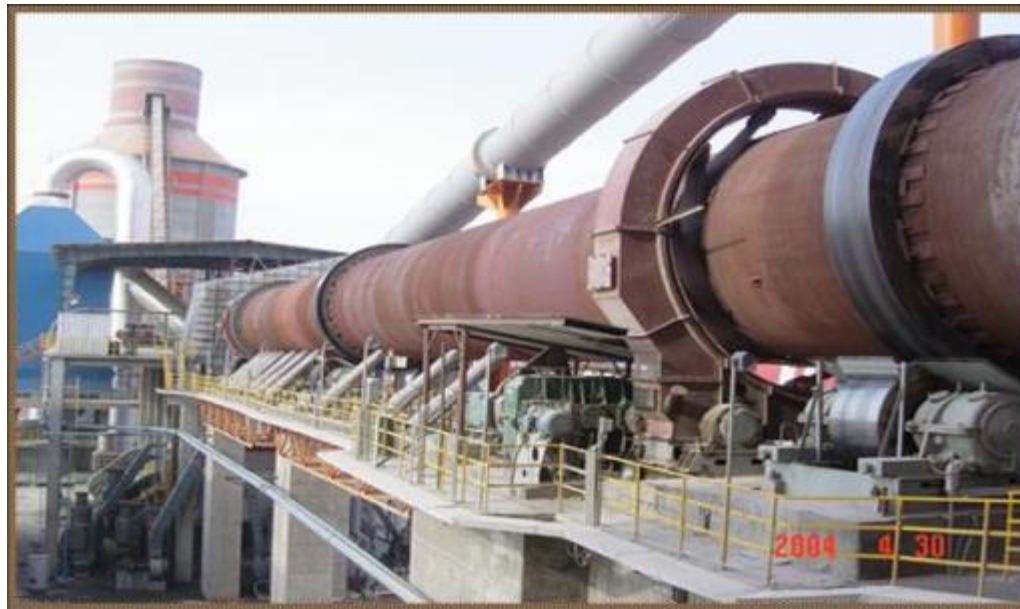
Three Pier Kiln
